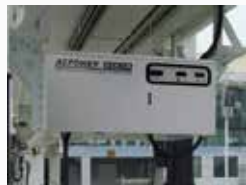
Airport Apron / Hangar
